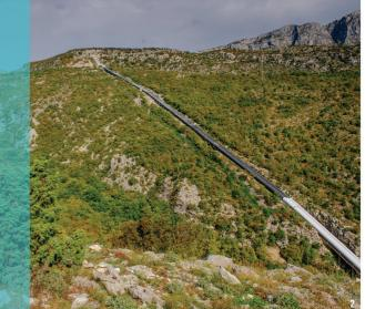
HPP 'Perucica' is impoundment derivation plant constructed not far from the Glava Zete which utilizes waters from the Niksicko field in order to generate electricity. It has been operating since 1960, and it got its name by the spring of Perucica situated in its vicinity.
